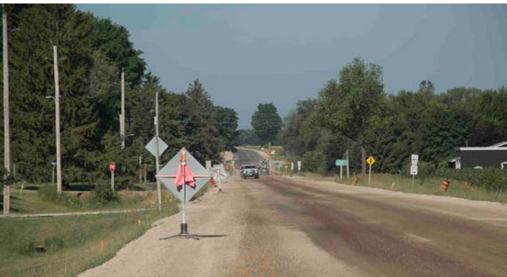
Construction continues on highway 87
